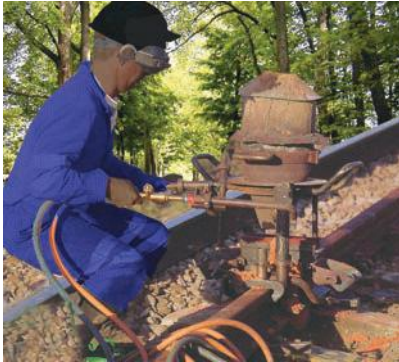
Figure 3.11 Thermit process for joining railway tracks
